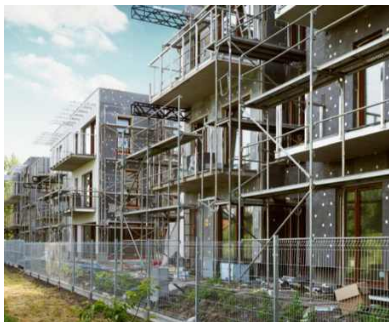
New sustainable housing projects in Spain
